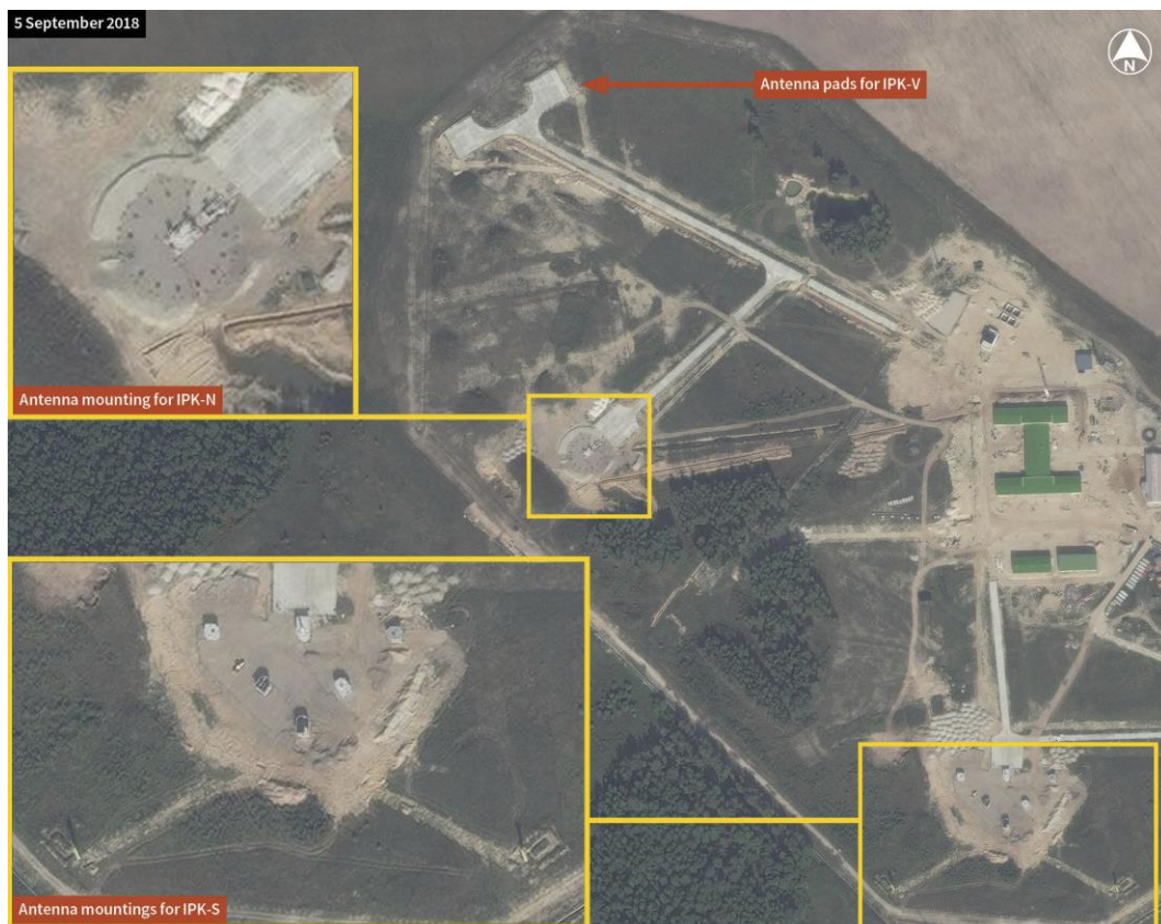
DigitalGlobe imagery showing a likely signals intelligence site under construction near Dubrovo, east of Moscow, including mountings and pads likely to be for three antennae complexes (IPK-V, -N, and -S) identified in online documentation related to the site.
